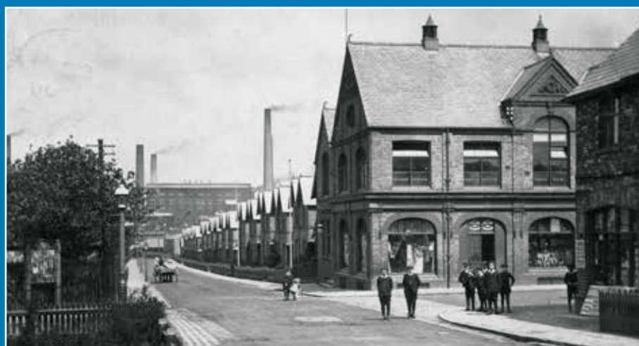
Brunner, Mond & Co. factory, worker cottages and Co-operative Society
